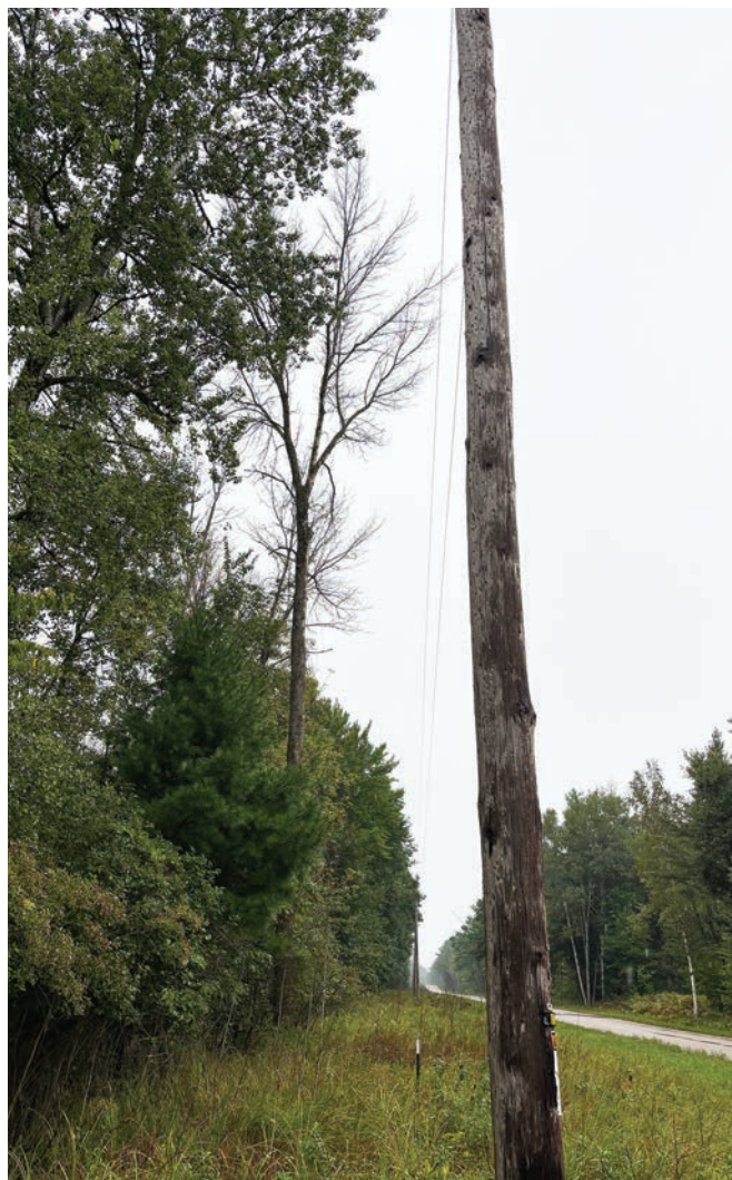
Dead ash tree located within the right-of-way that poses a risk of causing a power outage and requires removal.
