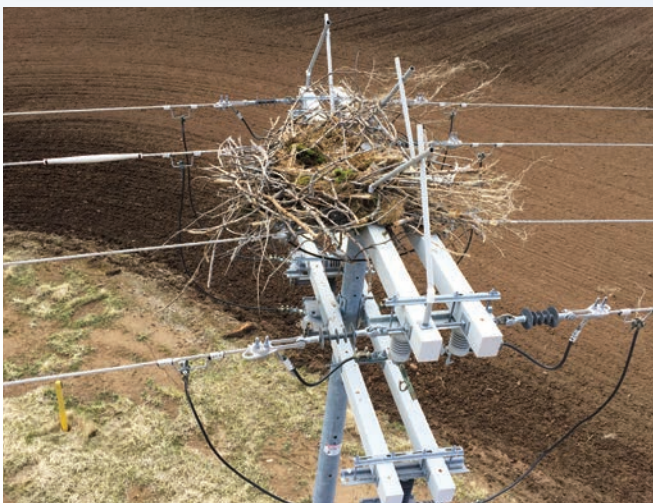
In 2015, osprey built a nest on our power lines. For safety reasons, the nest was removed and OEC put up a platform for the birds.
